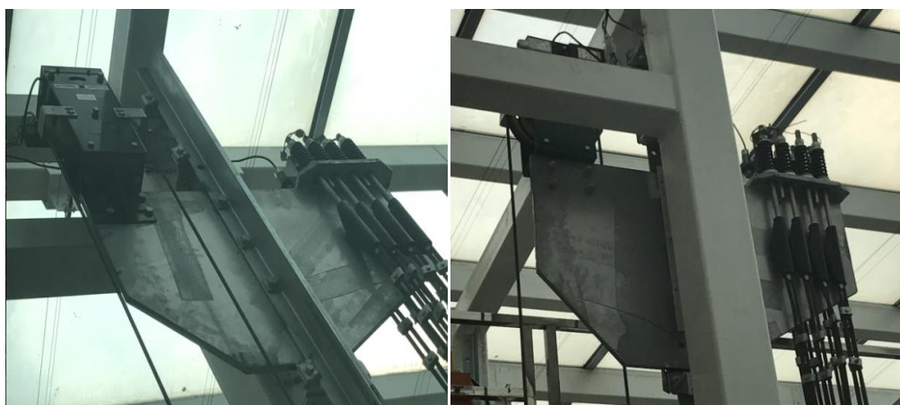
图 10-3 无机房限速器安装 Figure 10-3 Installation of governor without machine room
